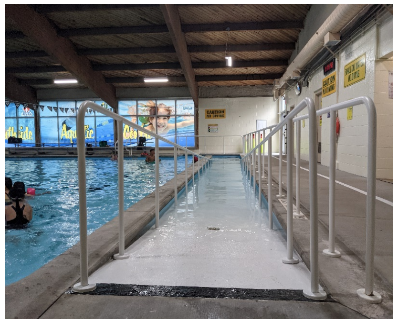
Southside Aquatic Centre pool and barrier-free entry ramp
